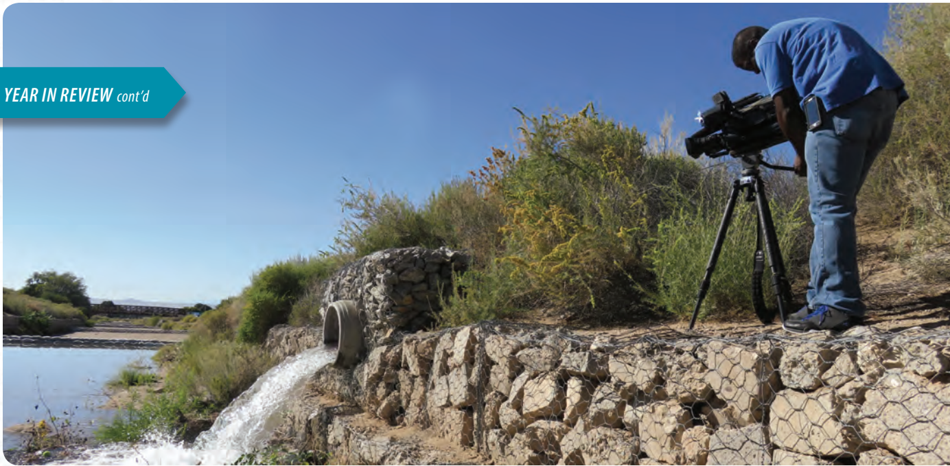
Above, a news cameraman films San Juan-Chama water flowing into the Bear Canyon Arroyo prior to its infiltration into the aquifer.
