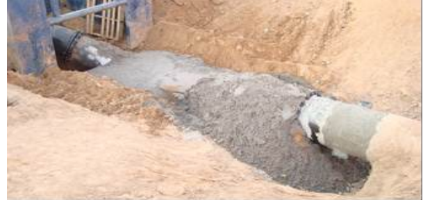
24" Concrete Cylinder Water Line
