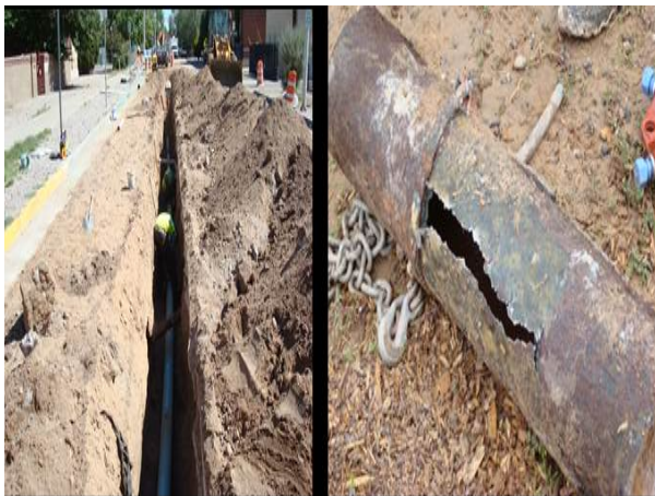
New 6-inch Waterline Installation
