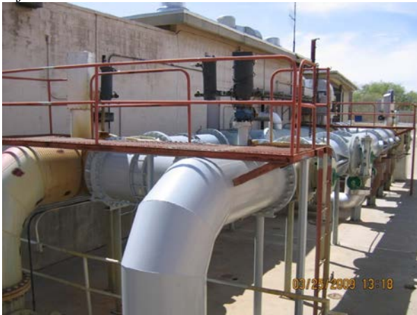
Lift Station #20 Force Main Header
