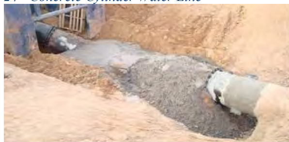
24" Concrete Cylinder Water Line
