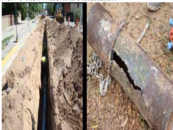
New 6-inch Waterline Installation
