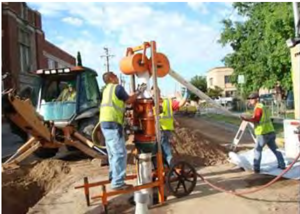
8-inch Sewer Lining Installation Project Downtown at 7th Street and Kent
