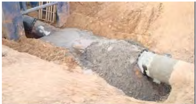
24" Concrete Cylinder Water Line Lowering and Relocation for a City Storm Drain Project in San Mateo NE
