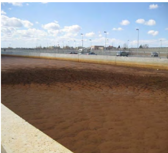
Sludge Drying Bed at SJCWTP
