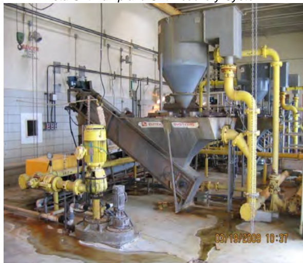
PTF Pista Grit Pump and Grit Recovery System
