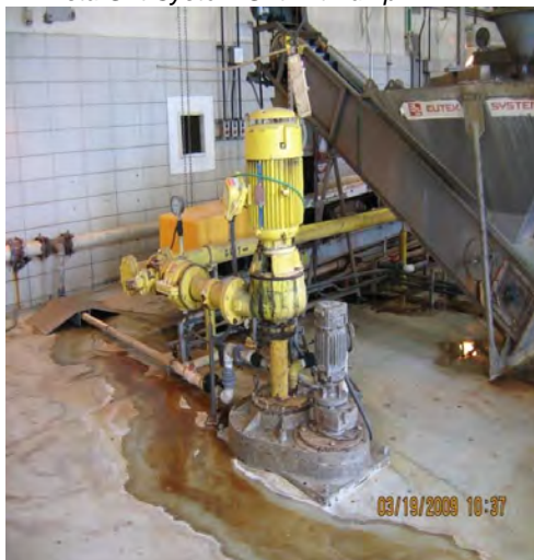
PTF Pista Grit System Grit Lift Pump
