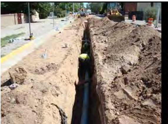
New 6-inch Water Line Installation
