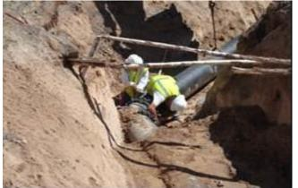
24" Concrete Cylinder Water Line Lowering and Relocation for a City Storm Drain Project in San Mateo NE
