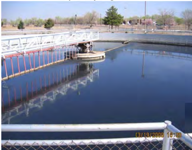
Uncovered Primary Clarifier generates odors
