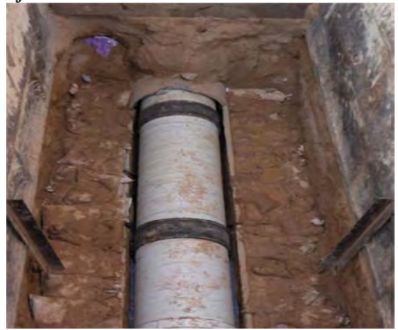
New 27-inch Sewer Line Slip-lined in the old 30" Concrete Pipe in Prospect NE west of Carlisle
