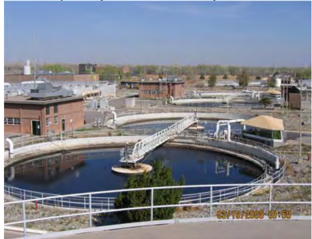
Primary Clarifiers to be covered for odor control
