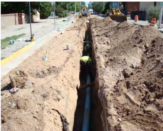
New 6-inch Water Line Installation
