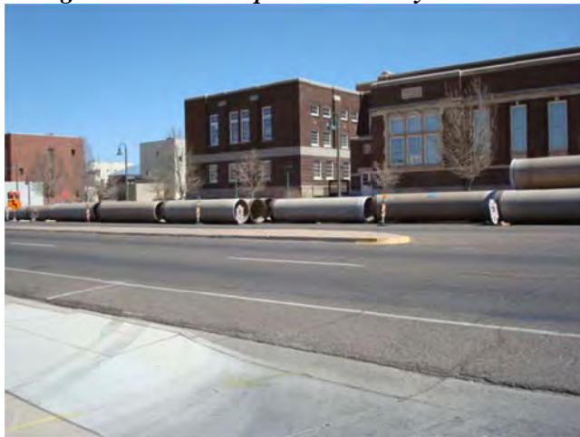
New 48" Sewer Line to be Slip-lined into an existing 54" Concrete Pipe in Broadway NE
