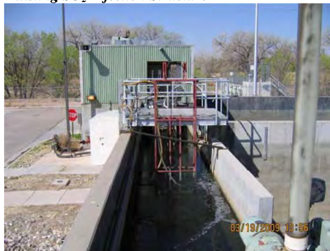
Existing SO 2 Injection Structure
