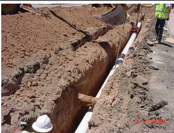
Old Cast Iron Waterline
