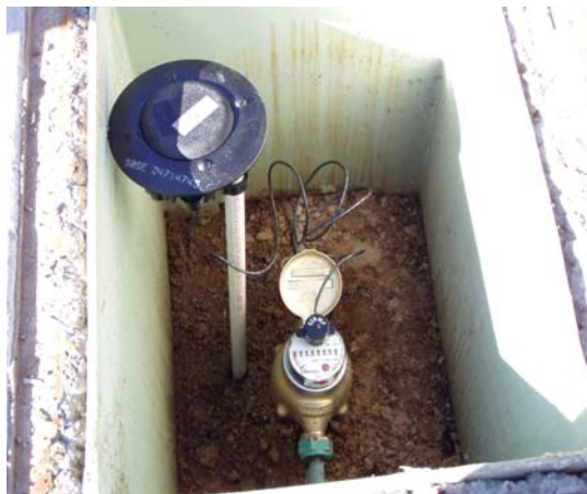
Installed Water Meter with AMR
