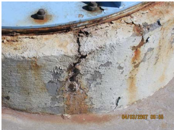
Failure at a mixer mount
