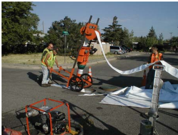
Cured In Place Pipe (CIPP) Setup
