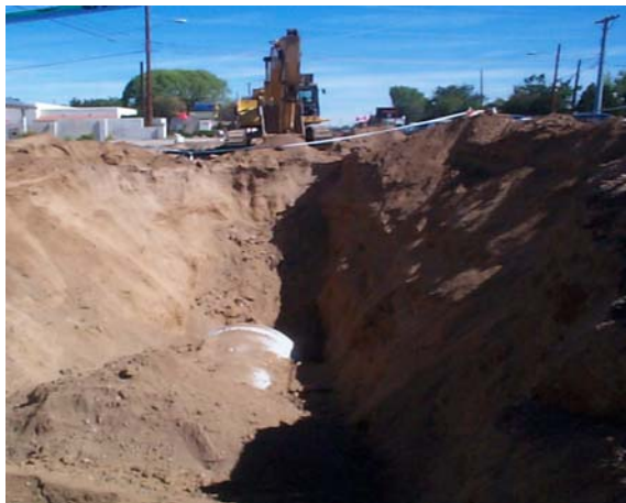
Backfilling Large Interceptor Sewer
