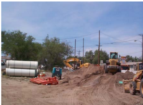
Large Interceptor Sewer Replacement
