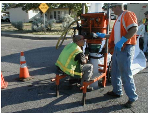
Cured In Place Pipe (CIPP) Installation
