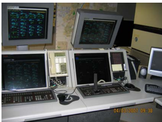
Control Room Bailey SCADA system
