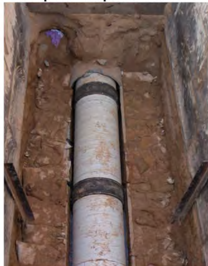
New 27-inch Sewer Line Sliplined in the old 30" Concrete Pipe in Prospect NE west of Carlisle
