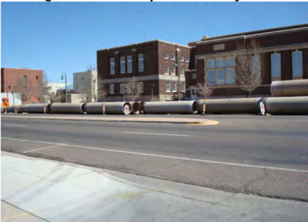
New 48" Sewer Line to be Slip-lined into an existing 54" Concrete Pipe in Broadway NE
