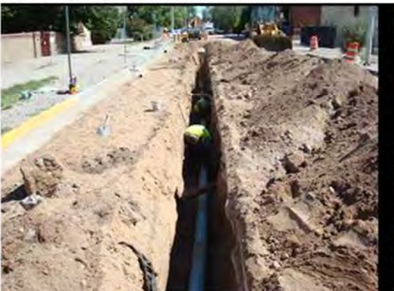
New 6-inch Water Line Installation
