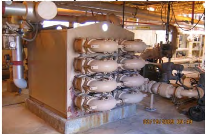
Digester Heat Exchanger for heating the sludge
