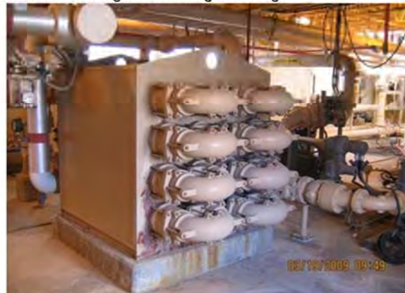
Digester Heat Exchanger for heating the sludge
