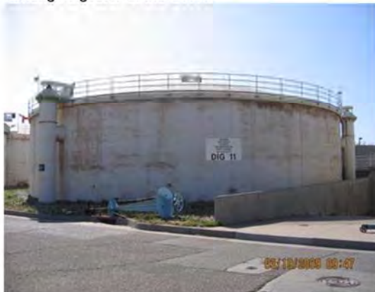
Existign digester at the SWRP
