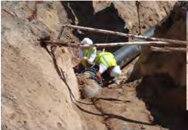
16" Ductile Iron Water Line Relocation for a City Storm Drain Project in Atrisco SW
