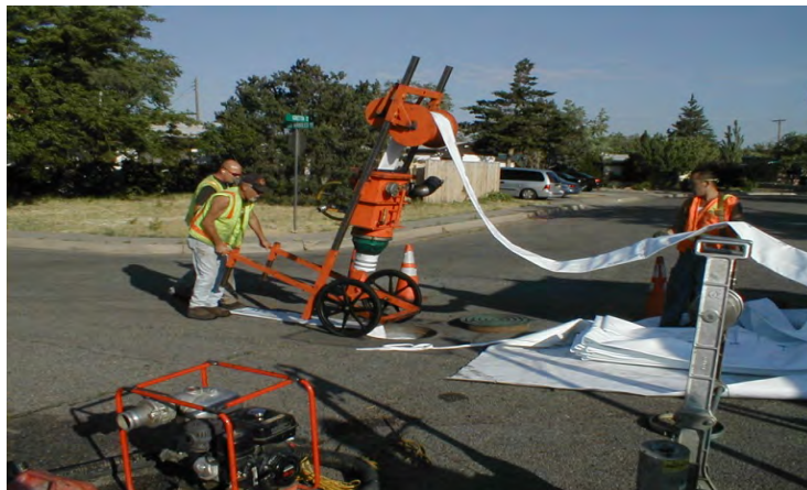
8-inch Sewer Lining Project on Los Arboles NE
