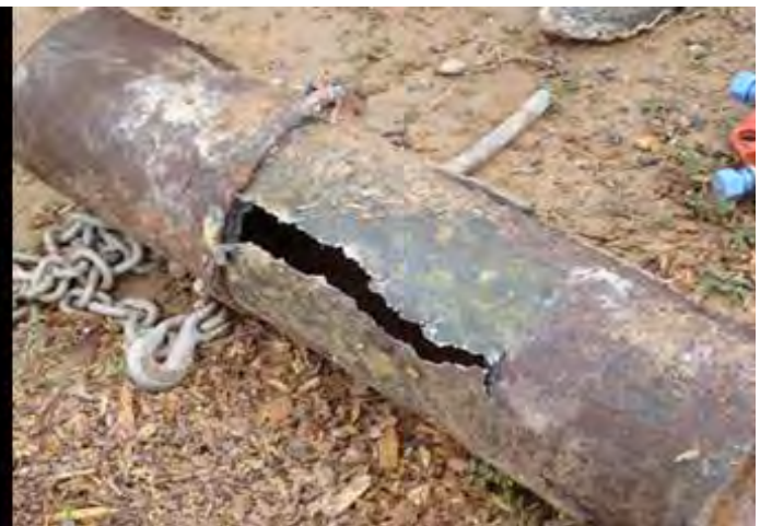
Old Steel Line at the Break Point
