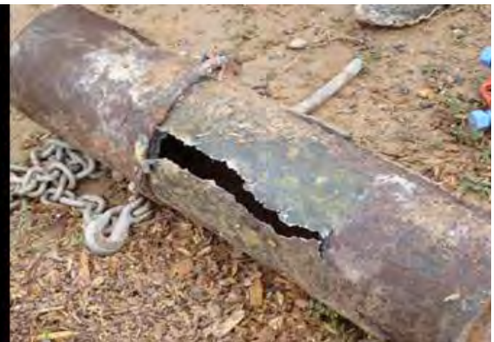
Old Steel Line at the Break Point
