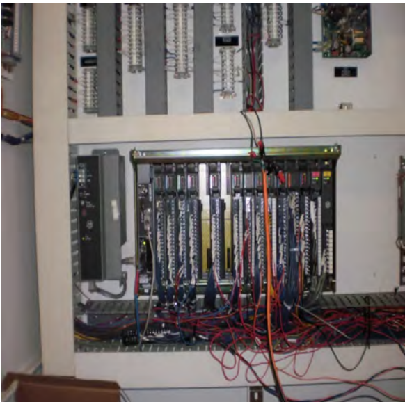
Sanitary Lift Station PLC-5
