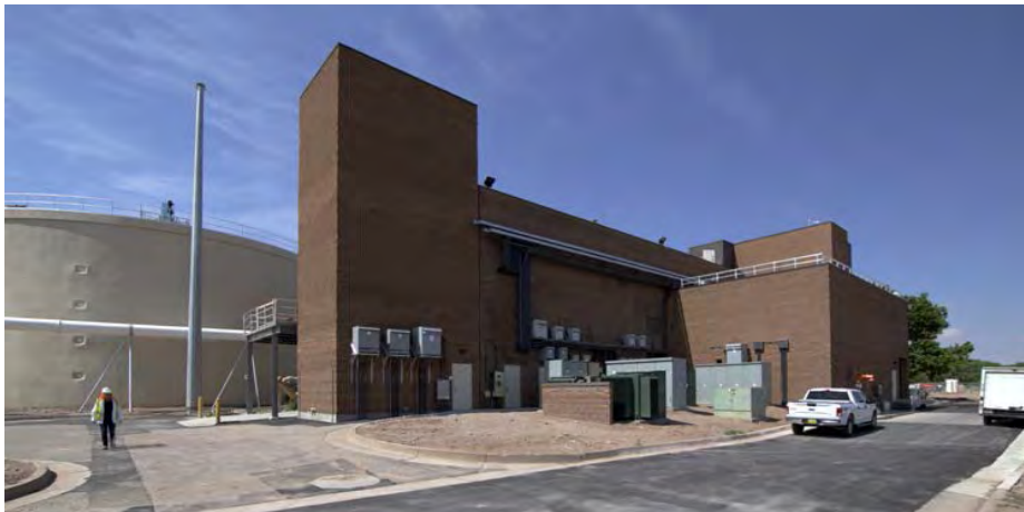
Renewed Solids Dewatering Facility
