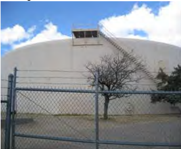
Existing Coronado Reservoir
