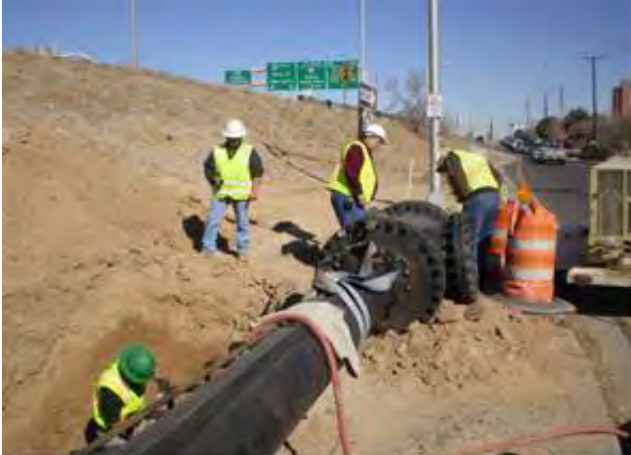
Large Valve, east of I-25
