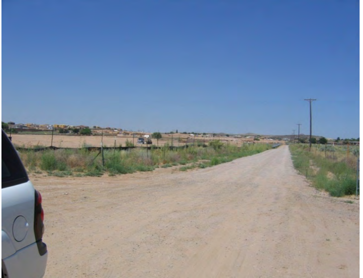
Lift Station #24 adjacent to new development
