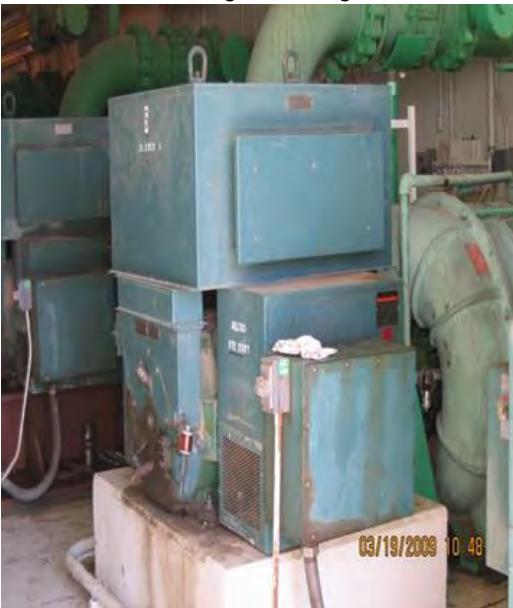
A Hoffman multi-stage centrifugal blower
