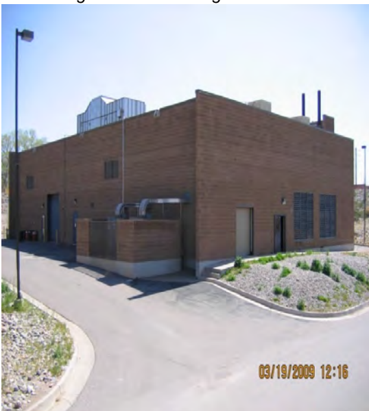
South Cogeneration Building
