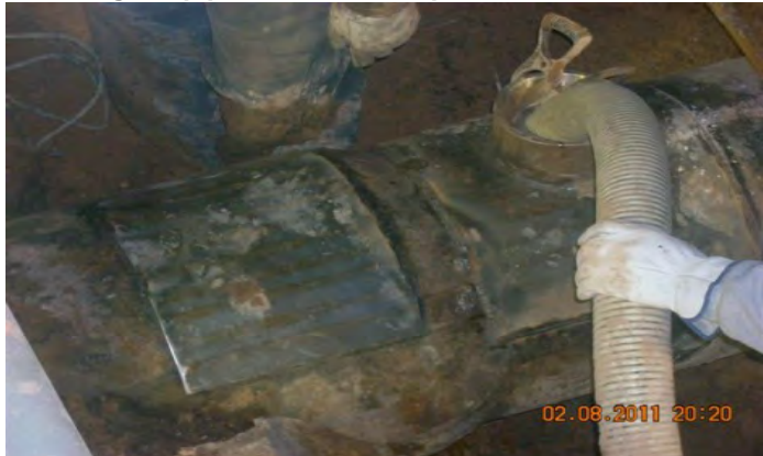
Patching the pipe with a welded plate
