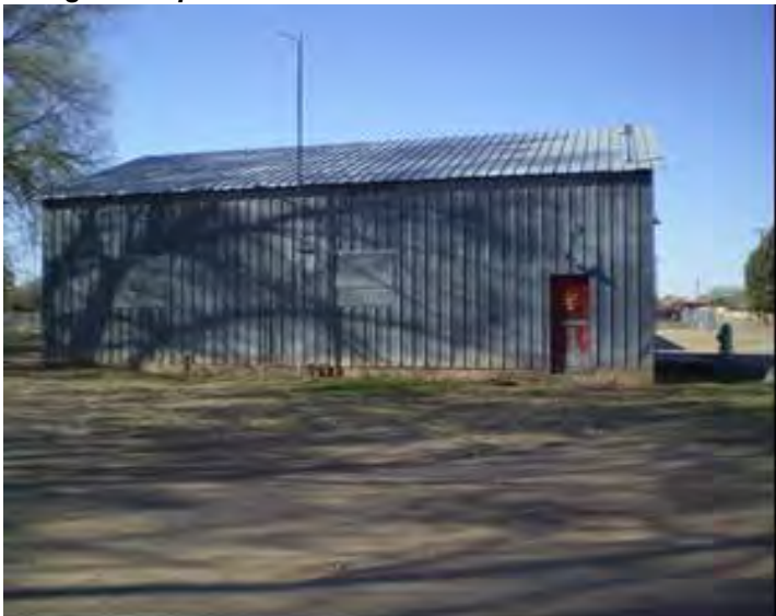
Griegos Pump Station - Exterior
