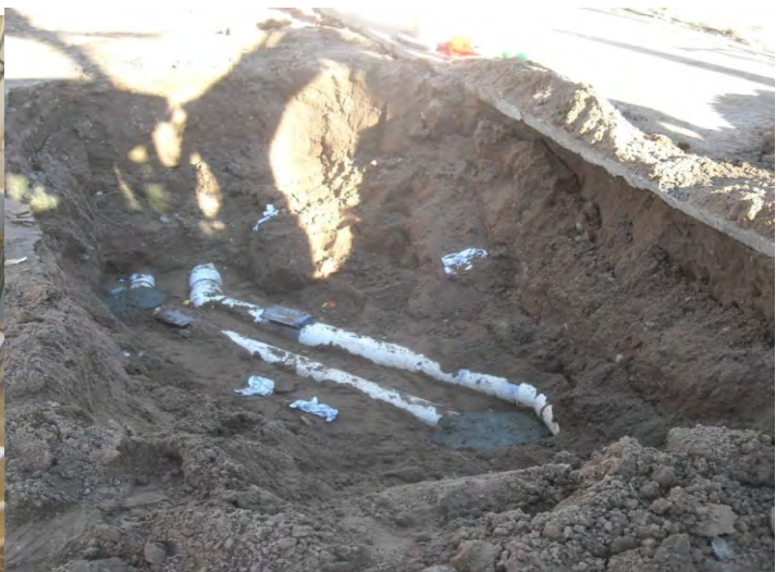
Force Main Repair - Station 68
