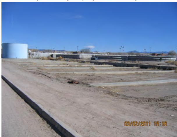
View of original sludge drying beds looking south
