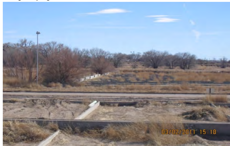
Sludge Drying Beds that were added in 1980's
