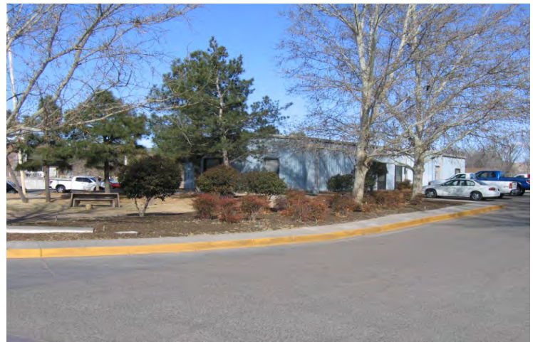
Metal Bldg from 1970's used for Staff Training
