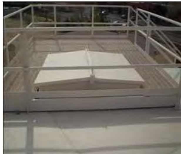
Secured Reservoir Hatch
