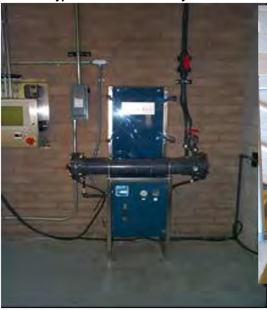
Sodium Hypochlorite Generator System
