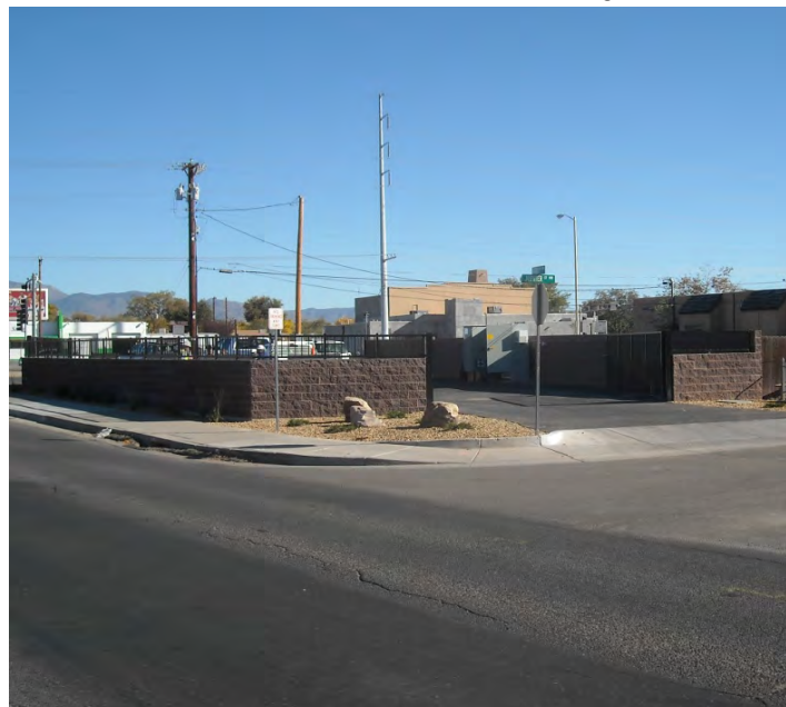
Odor Control Station 51. 2nd St. & Griegos
