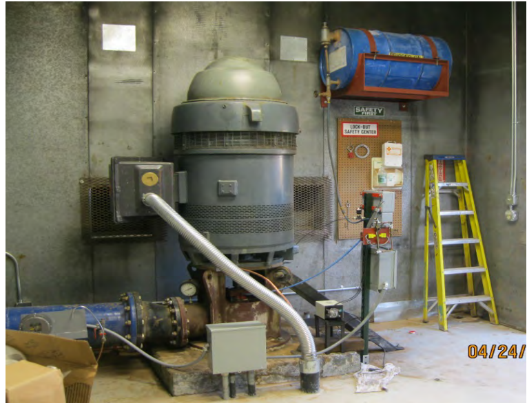
Corrales Well 1 - Electric driver replaced gas engine
