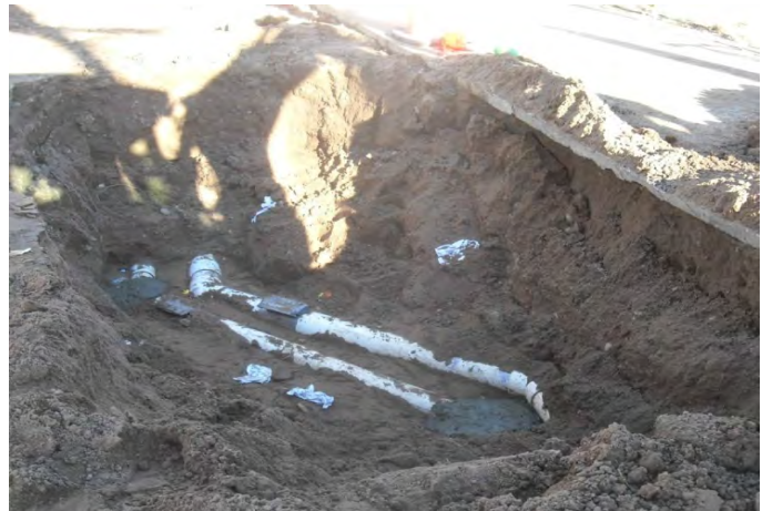
Force Main Repair - Station 68
