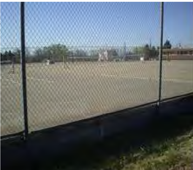
Charles Wells Reservoir - Tennis Courts on Reservoir Roof
