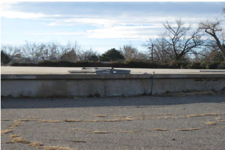
Charles Wells Reservoir - Concrete Tank
