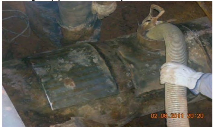
Patching the pipe with a welded plate
