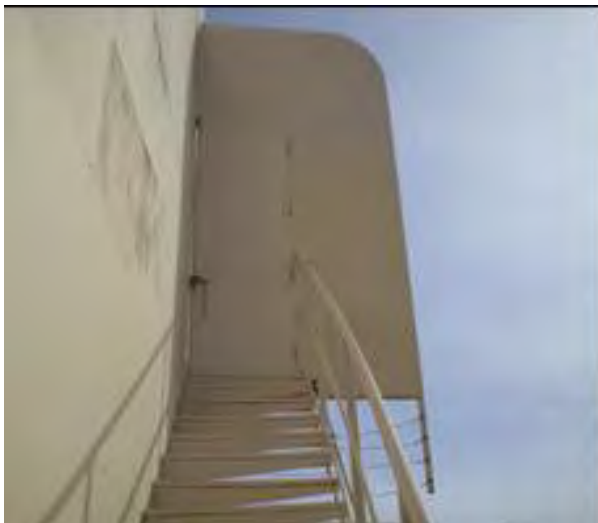
Reservoir Bulkhead On Staircase
