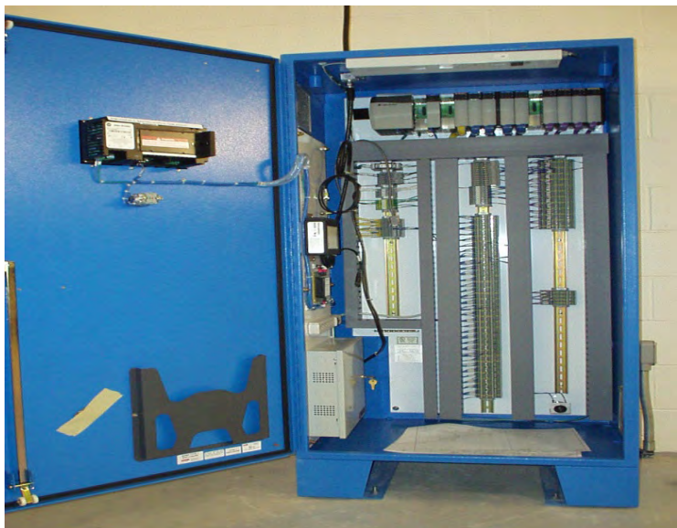
Typical ControlLogix PLC
