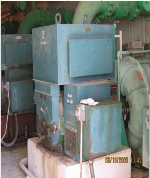
A Hoffman multi-stage centrifugal blower
