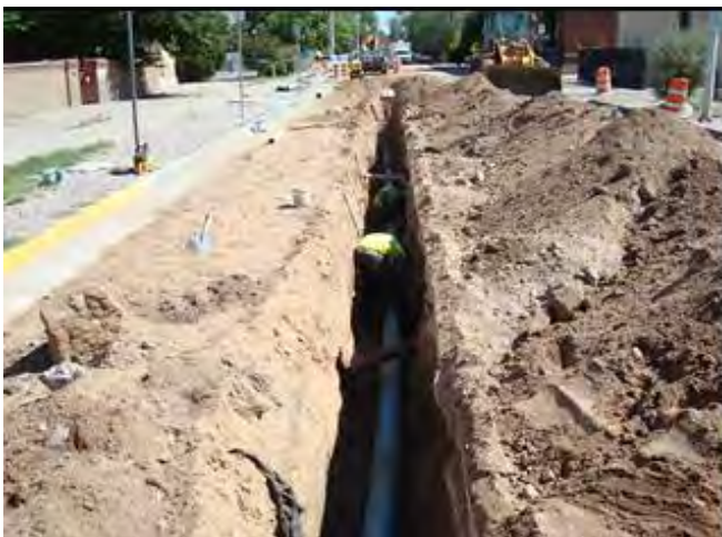
New 6-inch Water Line Installation
