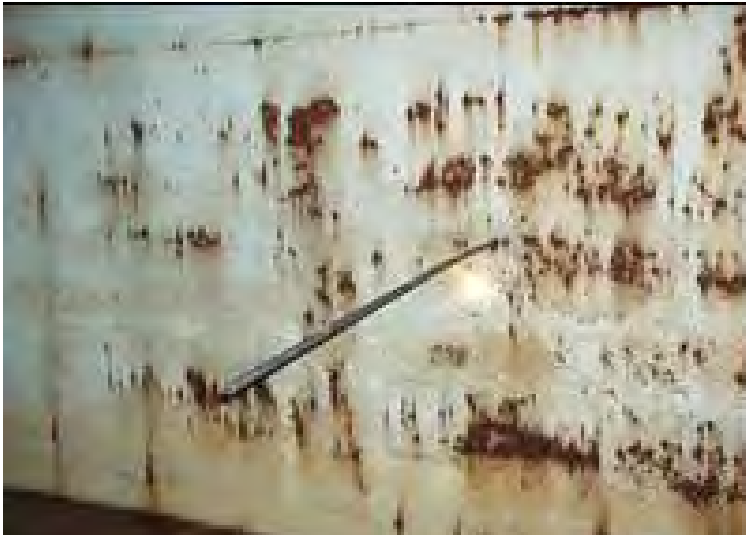
Interior of Volcano Cliffs Reservoir No. 1 Before Rehab
