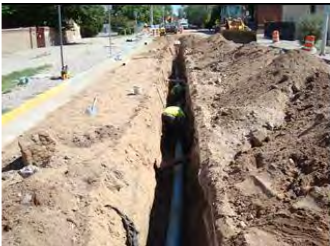
New 6-inch Water Line Installation
