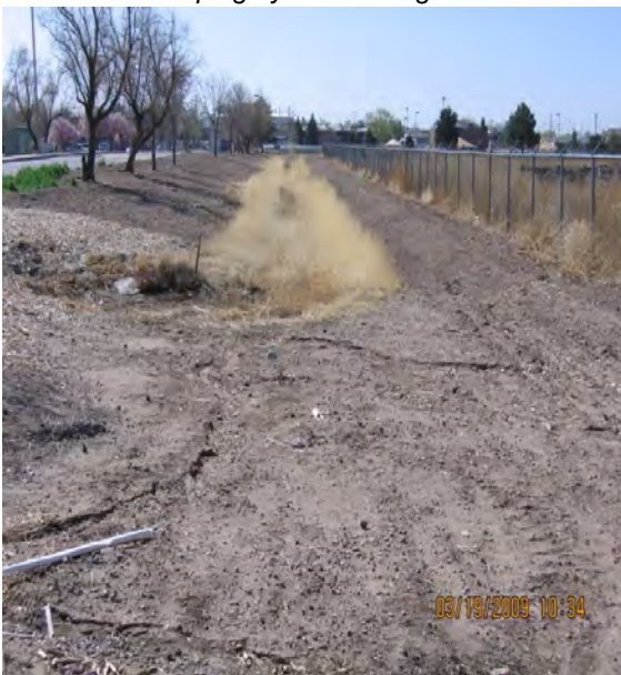
Failed Landscaping by Dewatering
