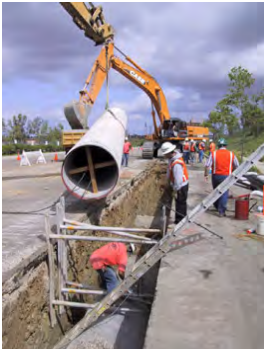
Typical Water Line Construction
