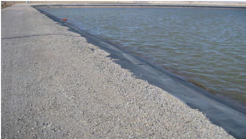
Edge of Settling Basin Embankment
